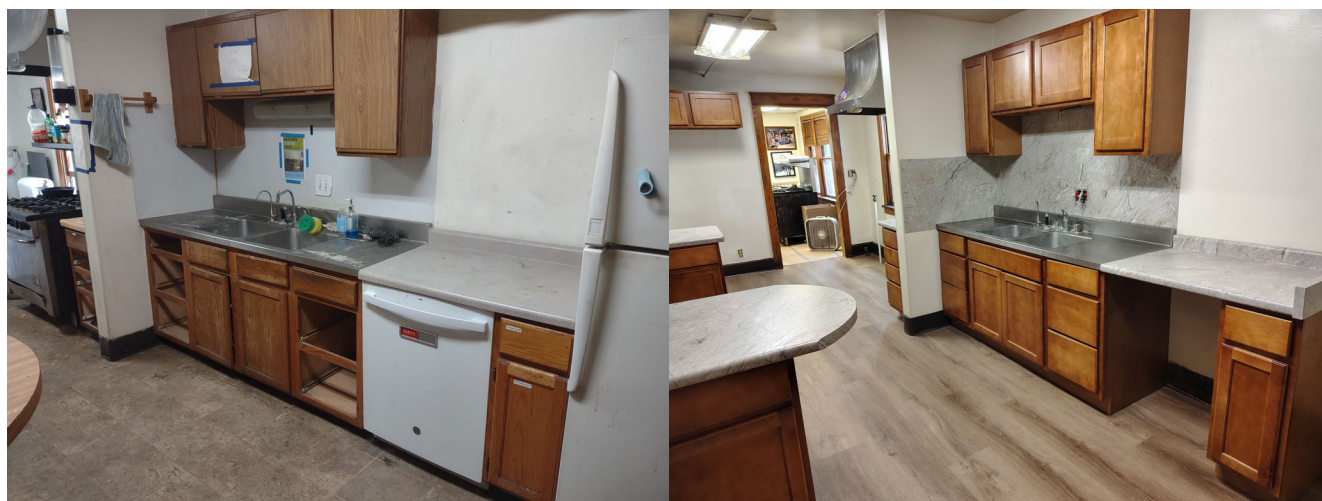
Photos of the kitchen sink area before (left) and after (right) replacement of the floor, lower cabinets, countertops, and backsplash. The metal sink basin was saved and cleaned up prior to reinstallation. New cabinets were also added above the two refrigerators for additional storage.
