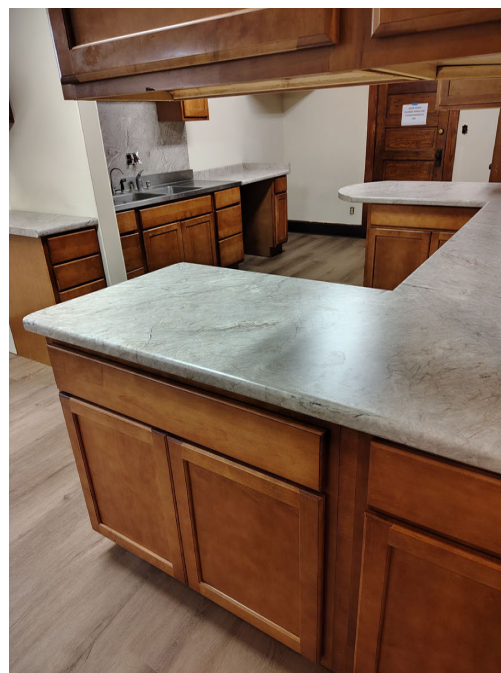
Close-up photo of new lower cabinets and countertops. The cabinets match the double-sided design of the previous, and match the design and color of the upper cabinets.
